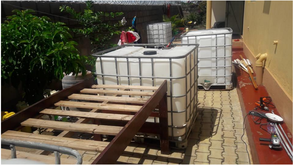
Preparing the wooden support structure for the grow beds.
