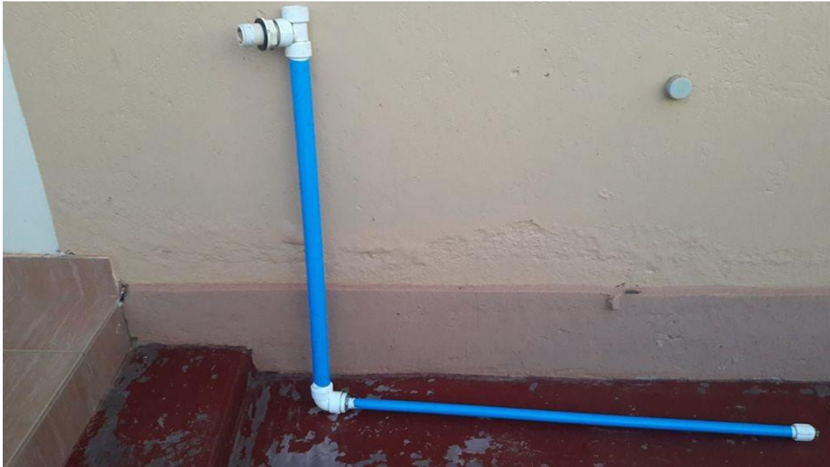
Solids Lift Overflow.
