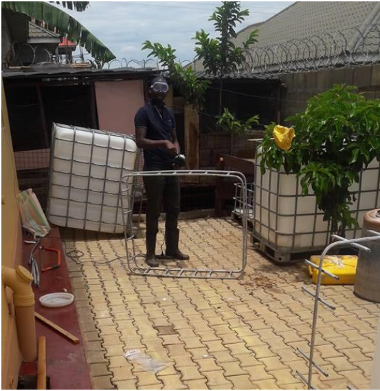
Cutting the IBC tank metallic frames using a grinder.
